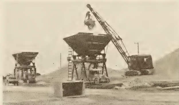
FIGURE 2.—TWO BINS WITH STRAIGHT DRIVE THROUGH BOTH STOCK PILES ON OPPOSITE SIDES OF TRACK. CRANE WORKING ON A RAMP MADE OF COARSE AGGREGATE
